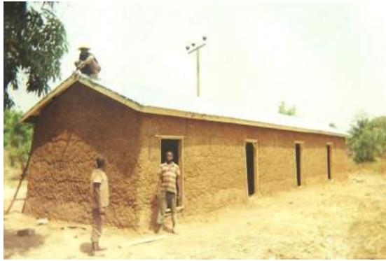
Finishing off a building – CHIPS base, Ghana
