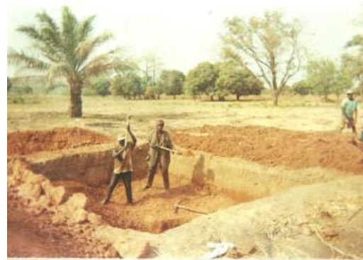
Work begins on the CHIPS base in Ghana
